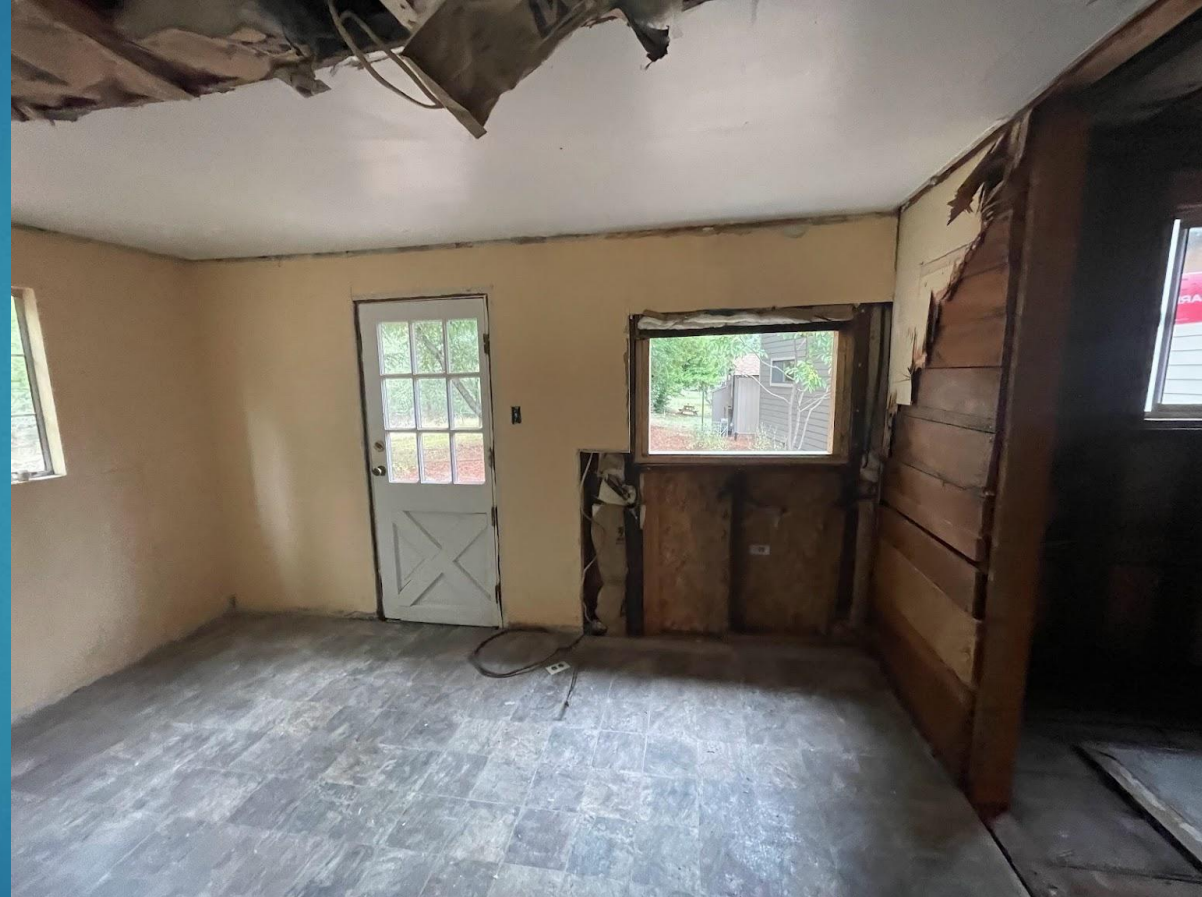
Window prepped for dining room area
