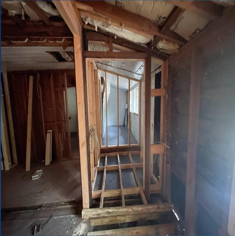
Framing for the mandir area
